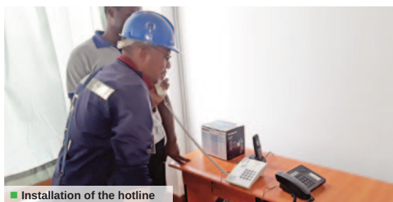
Installation of the hotline
